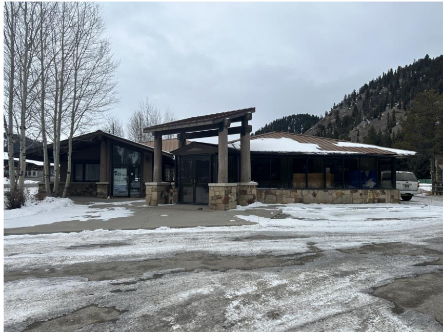
An exterior view of the commercial building located at 55 Lone Mountain Trail. Photo taken on January 4, 2024 by Dan Wheeler.
